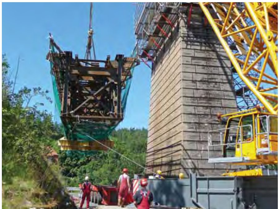
Brückenaushub in Angelroda
